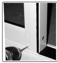
On bottom of the interlock, use screws (12X8) to secure bottom interlock to the sill both inside & outside.
