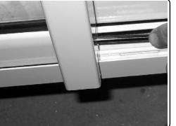
7- Place the sliding panel into frame on the inside. - If required, Adjust the rollers from either end of sliding panel with phillips screwdriver.
