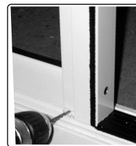
5-On top of the interlock, lift the Top fix block to touch the Head frame. Use screw (12X8) to secure it to frame.
