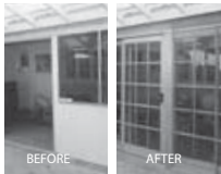
Stegbar Installation Service
